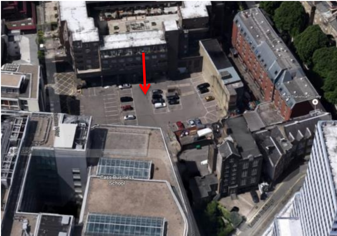
View of site looking from the East to the West
