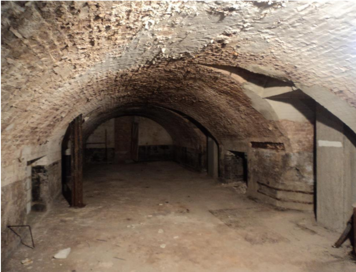
Internal view of existing grade II listed vaults at upper basement level.
