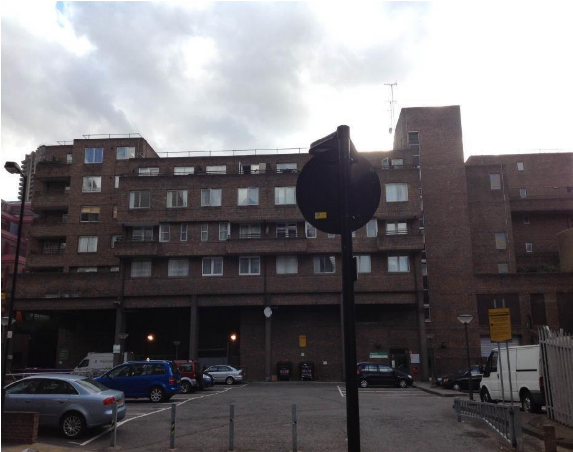
View of the rear of Shire House facing onto the application site from Lamb's Passage
